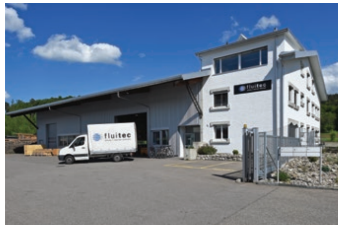
Fluitec in the year 2015
